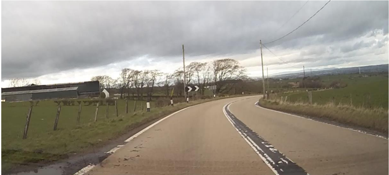
Northbound view of location of the slight injury collision on 16 July 2020
