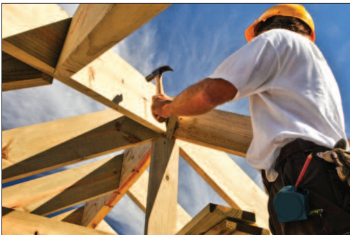
Timber roof construction
