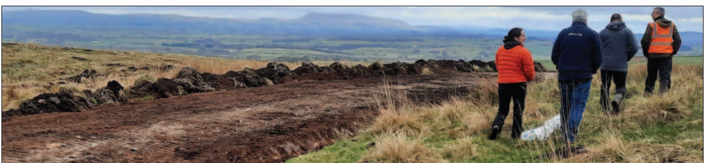
Road building foundations
