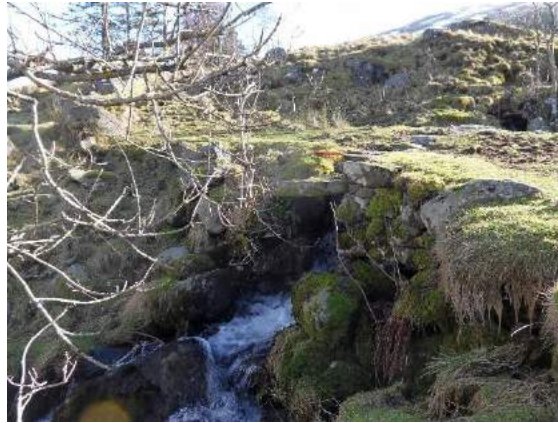
Photo 4.9: Surviving clapper bridge MM18f crossed by track MM18b, looking south-east
