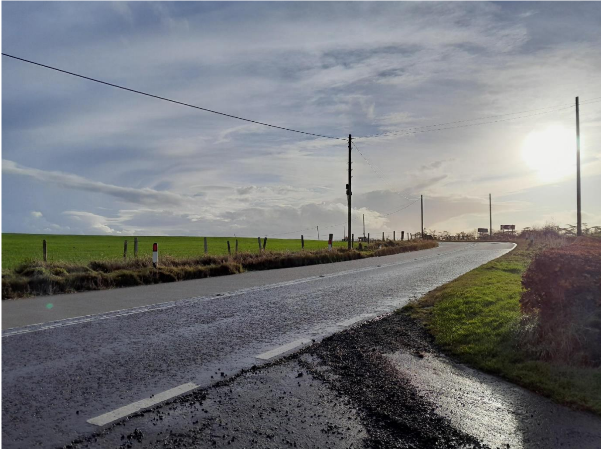
Figure 6. Sight line looking southwest along the A723. A 5-metre buffer has been created around this sight line and the tree design in the field to the east of the A723 has been reduced accordingly.
