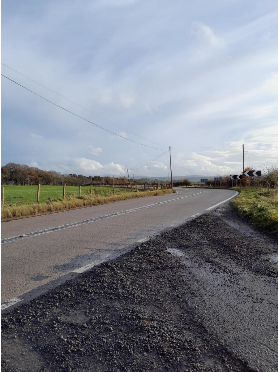
Figure 4. Sight line looking south along the A723. A 5-metre buffer has been created around this sight line and the tree design in the fields to the east and west of the road have been reduced accordingly.
