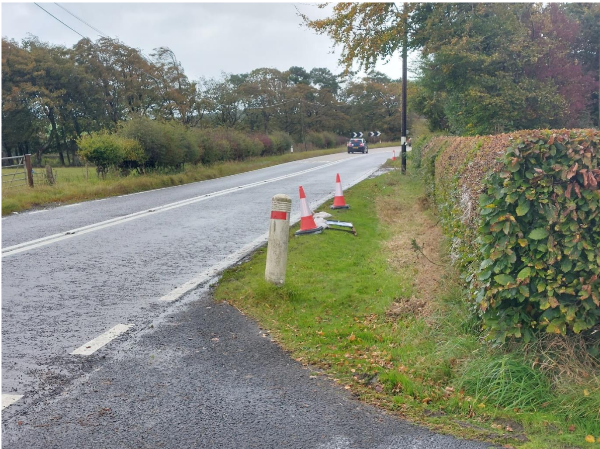
Figure 1. A723 looking south. Sight line to bend only. Tree planting will not affect this sight line.
