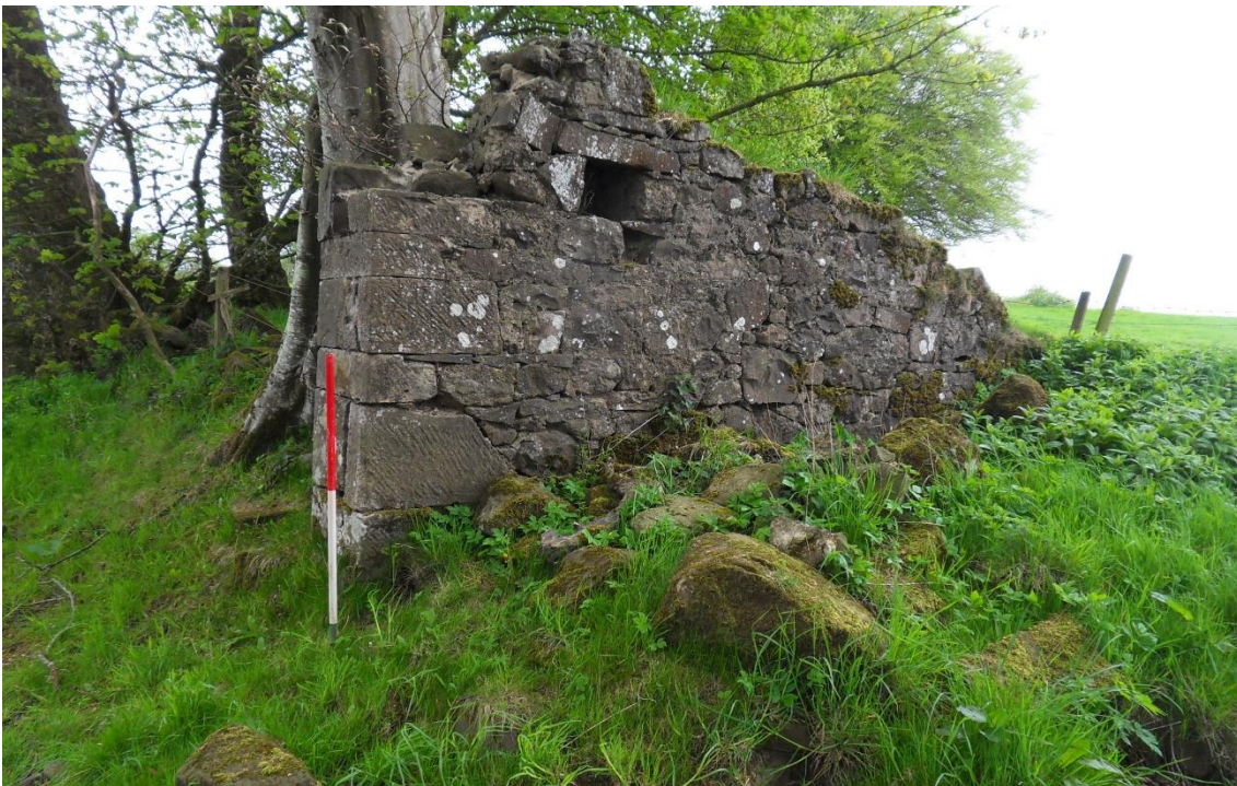
Photo 5.5: View south-west showing southern gable of High Barn farmstead (MM06)
