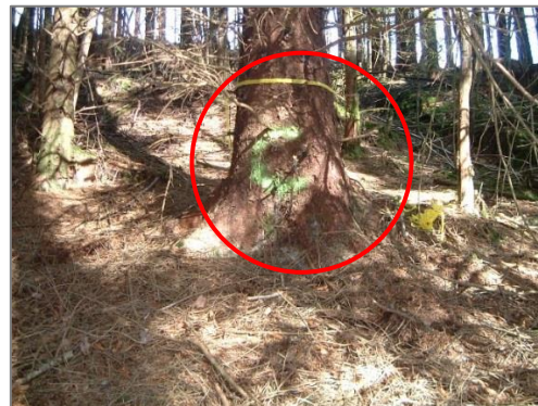
Boundary marking at ground level due to heavy branching. Note the use of Tape & Spray Paint
